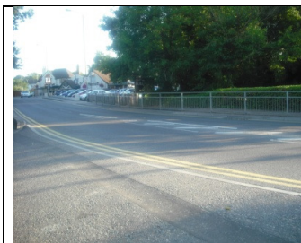
Railings on southern approach
